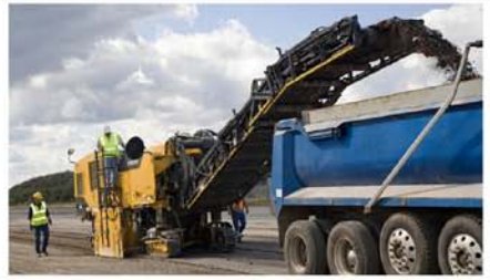
Road Surface Asphalt Milling
