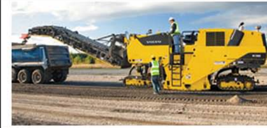
Road Surface Asphalt Milling
